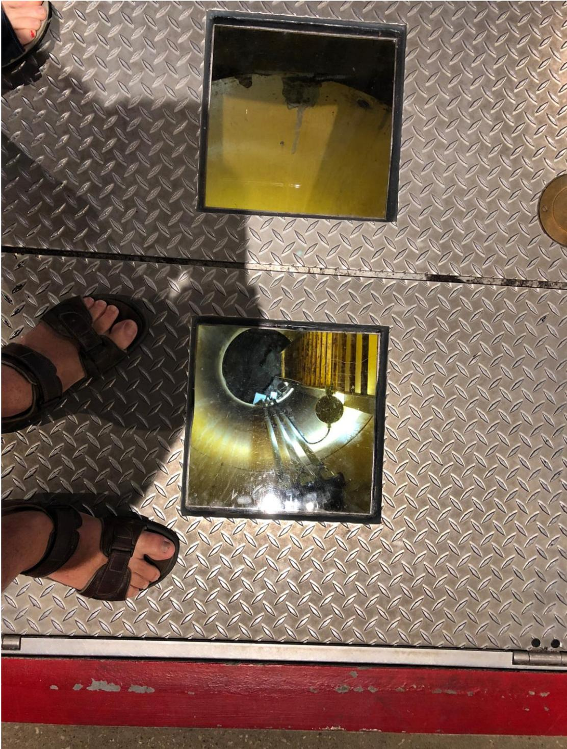
They have left an inspection shaft so they can keep an eye on the erosion that is still happening under the central cone of the museum exhibition.
