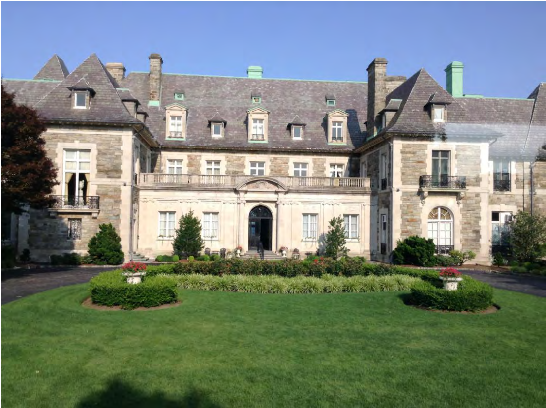
Another Mansion in Warwick, Rhode Is.
